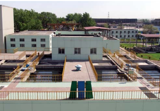
高效澄清池 High-efficiency Clarifier
