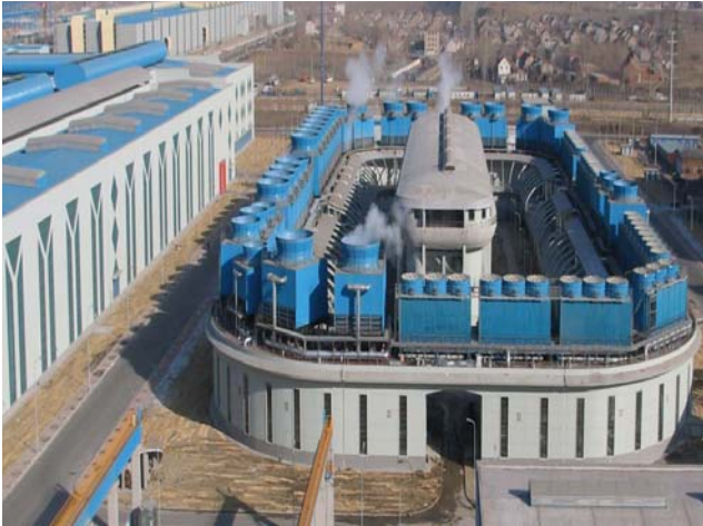
椭圆形集中水处理设施 Elliptic centralized water treatment facility
