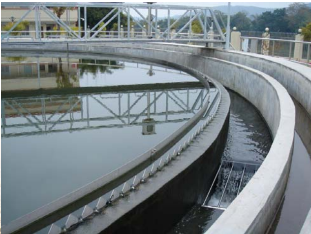
污水处理二沉池 Secondary sedimentation tank for waste water treatment
