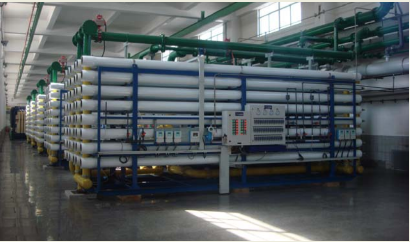
污水深度处理超滤膜组件 Ultrafiltration Membrane Components for Deep Waste Water Treatment
