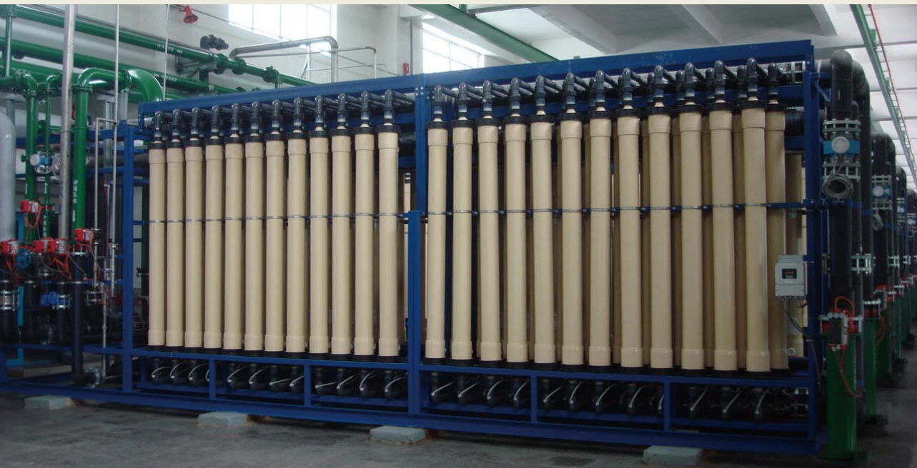
污水深度处理超滤膜组件 Ultrafiltration Membrane Components for Deep Waste Water Treatment
