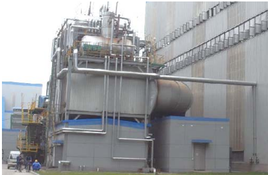
首钢京唐580m²环冷机余热利用设施 Residue heat utilization facility for Shougang Jingtang 580m² annular cooler
